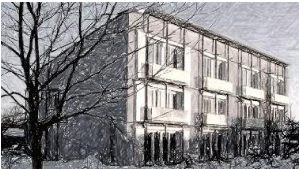
Figure 1: The Kranichstein passive house is a solar-optimised row house with 156 m 2 living space on 2.5 floors
